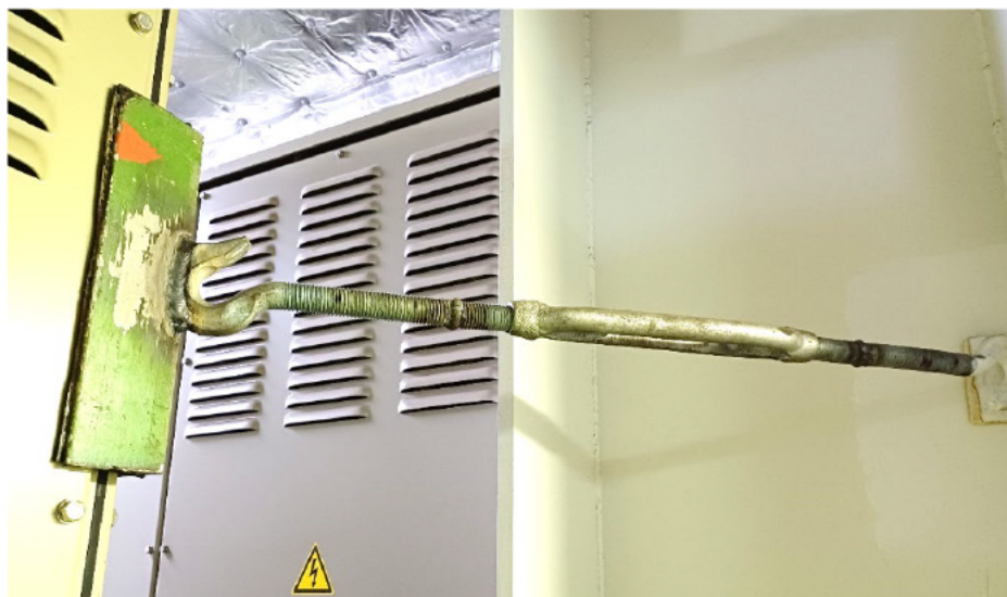
Cargo chain turnbuckle, welded to angle iron, and wedged between the number 1 step-down transformer (left) and a steel beam (right).
