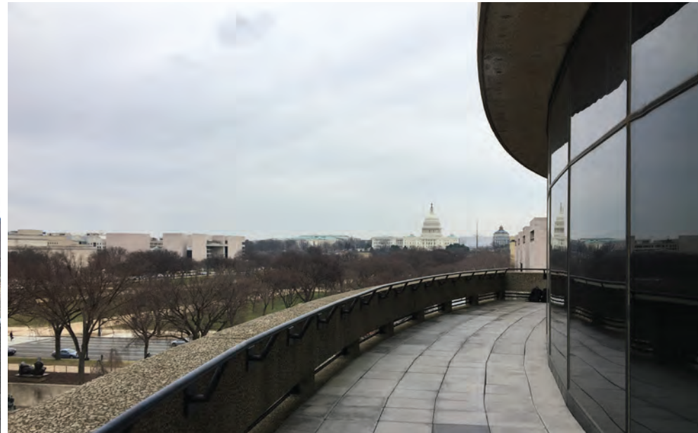
Balcony pavers and rail
