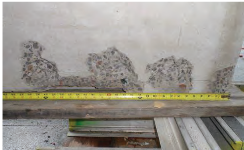
Concrete panel intentionally chipped for anchorage installation
