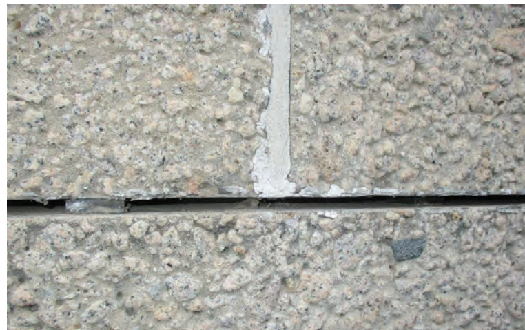
Hard plastic shims (ovals) between small panel (above) and large panel (below)
