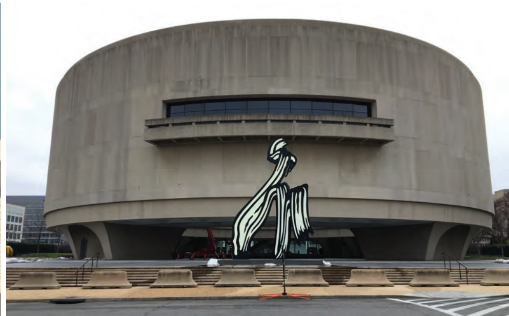
North facade precast panels
