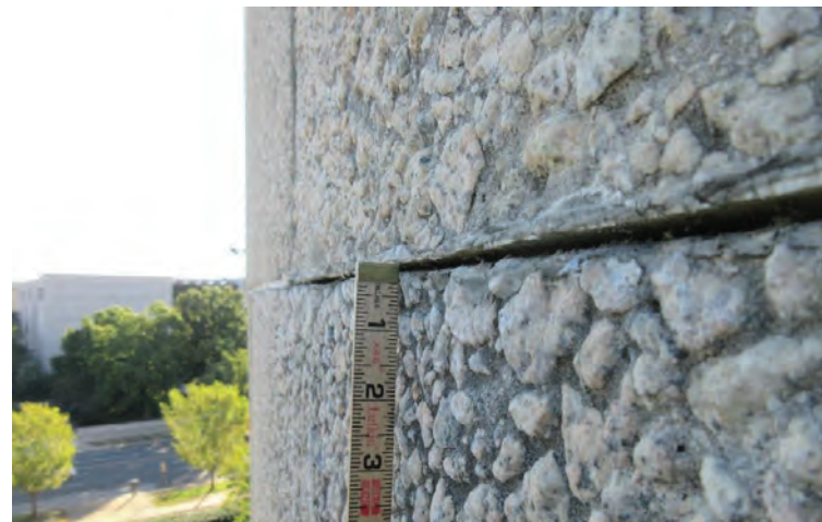
Large panel bearing on small panel below and uneven spacing between panels
