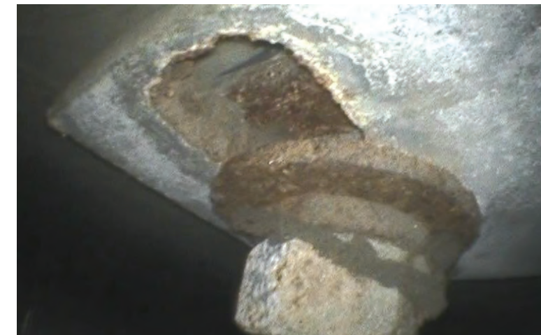
Flame cut slotted hole in strap plate connection to backup wall
