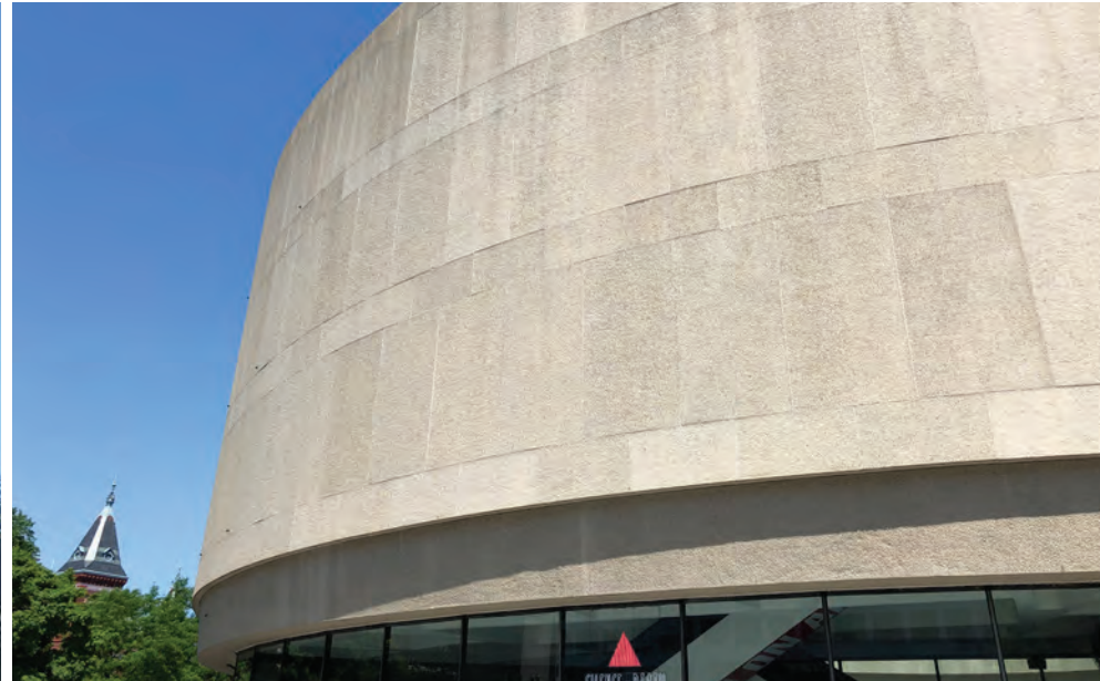
South facade precast panels
