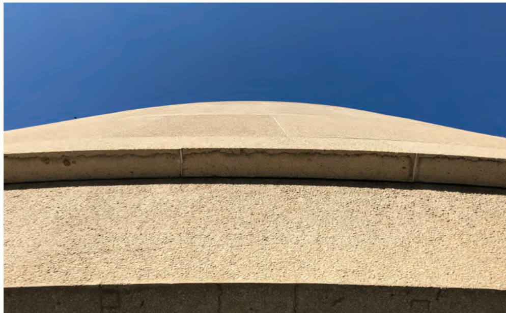
Facade soffit panels
