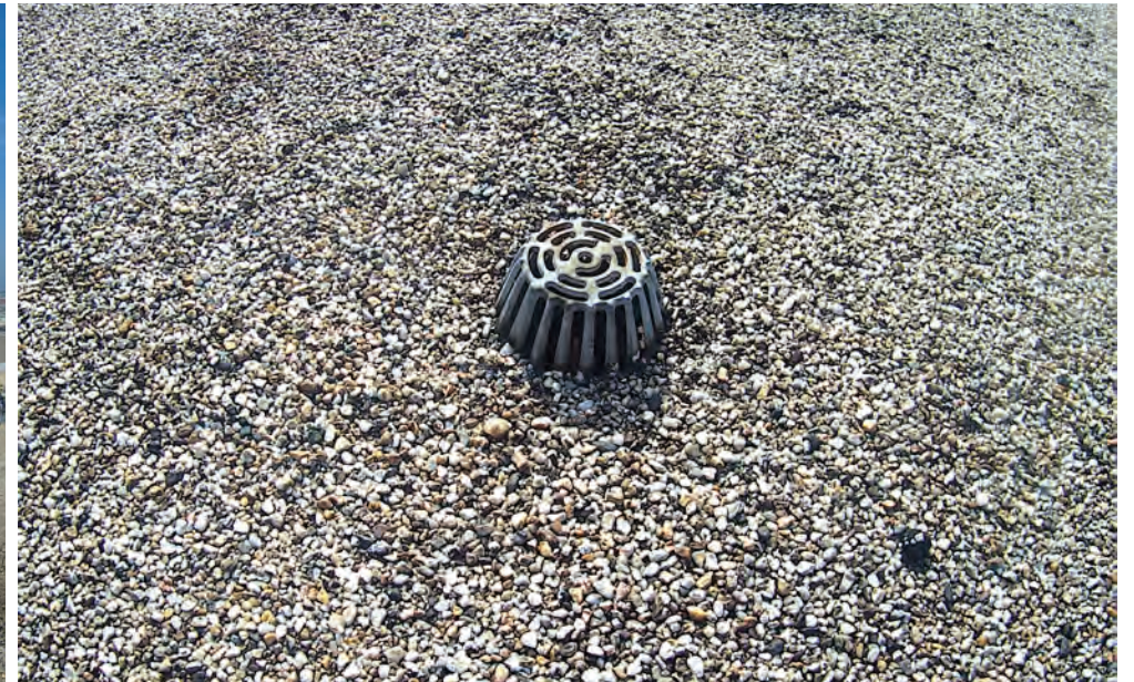
Roof assembly and roof drain
