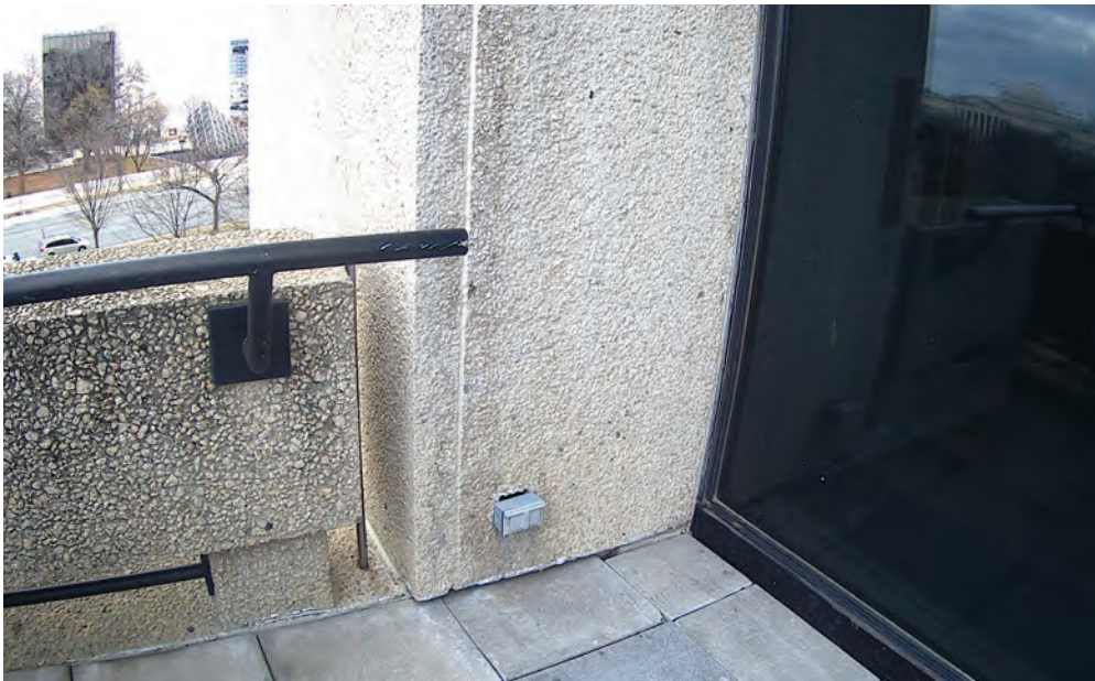
Balcony rail and facade panel
