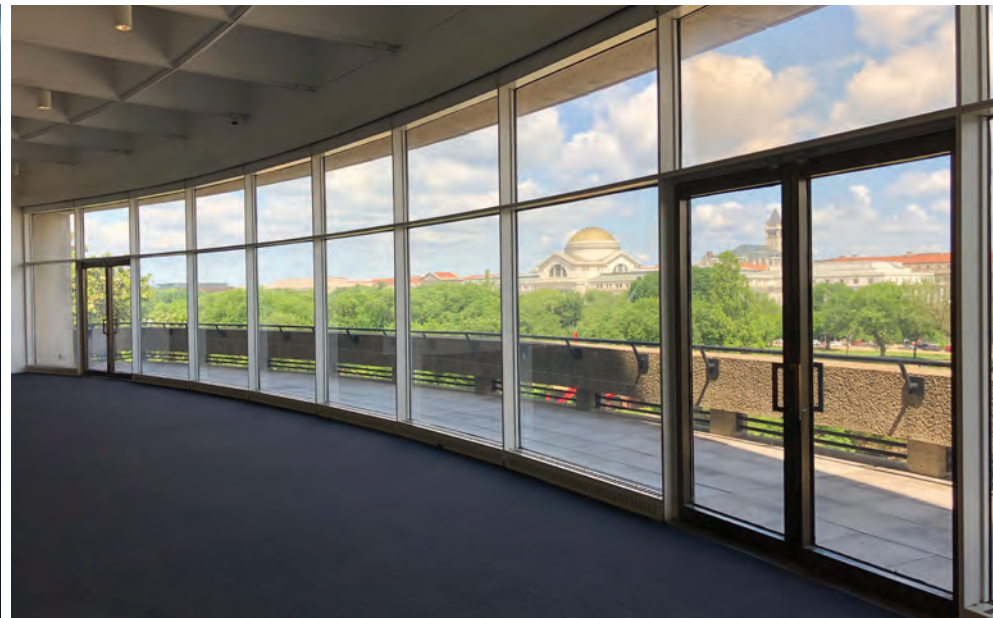
Balcony glazing interior side
