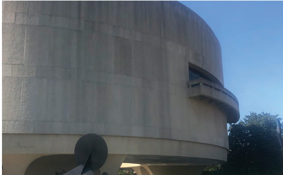
East facade precast panels
