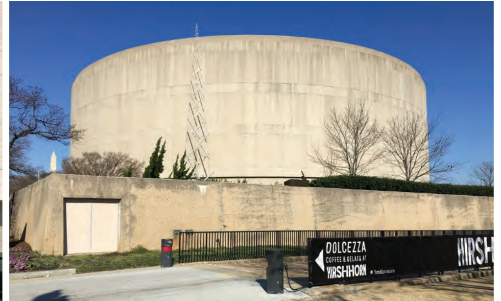
East facade precast panels
