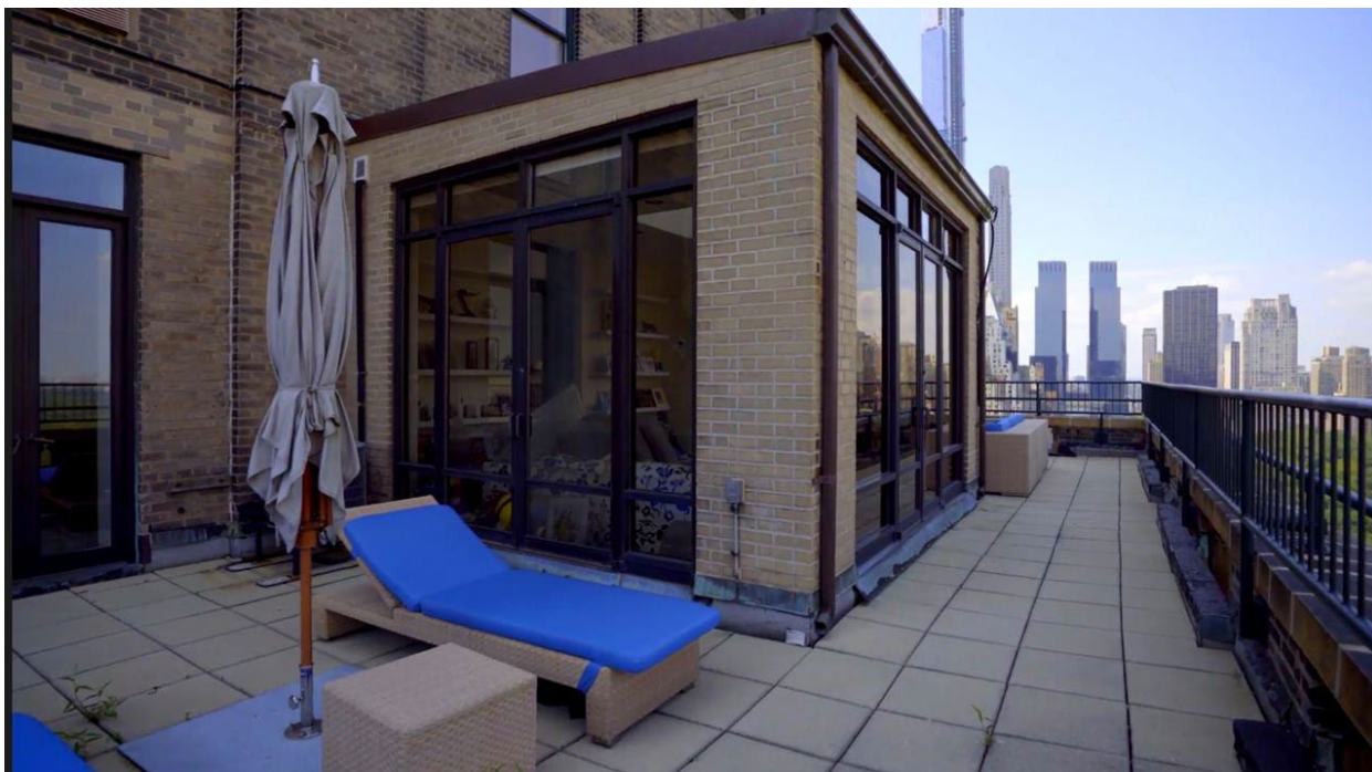
Figure 2: Westerly-facing views of terrace (pre-scaffolding)
